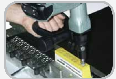
Electric Powered Rivet Driver Installation
