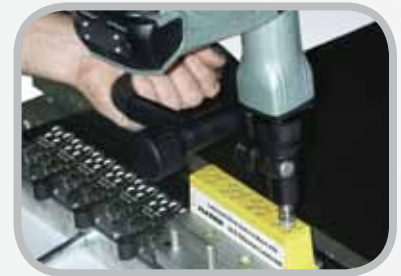
Electric Powered Rivet Driver Installation
